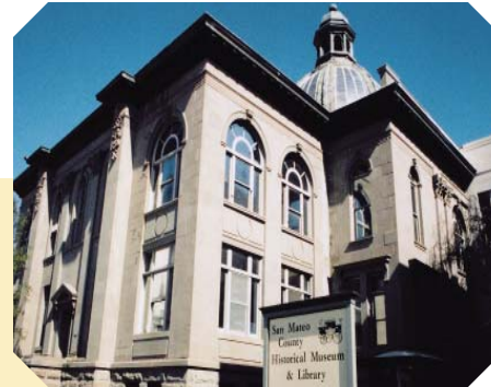
1999 San Mateo County Historical Association moves into Courthouse - Entrance to Museum? Hidden side door on Hamilton Avenue
