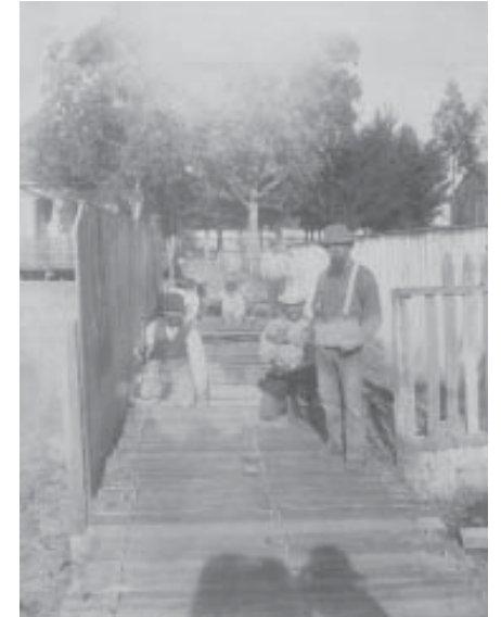
Building a Wooden Sidewalk in Redwood City
